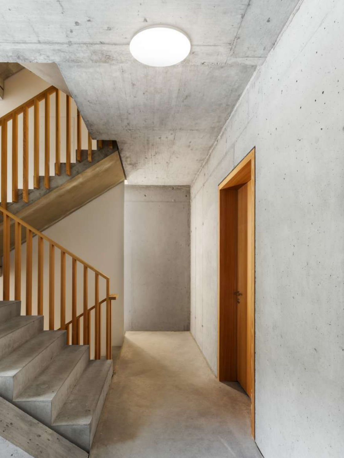
INDOOR - CEILING FIXTURES
