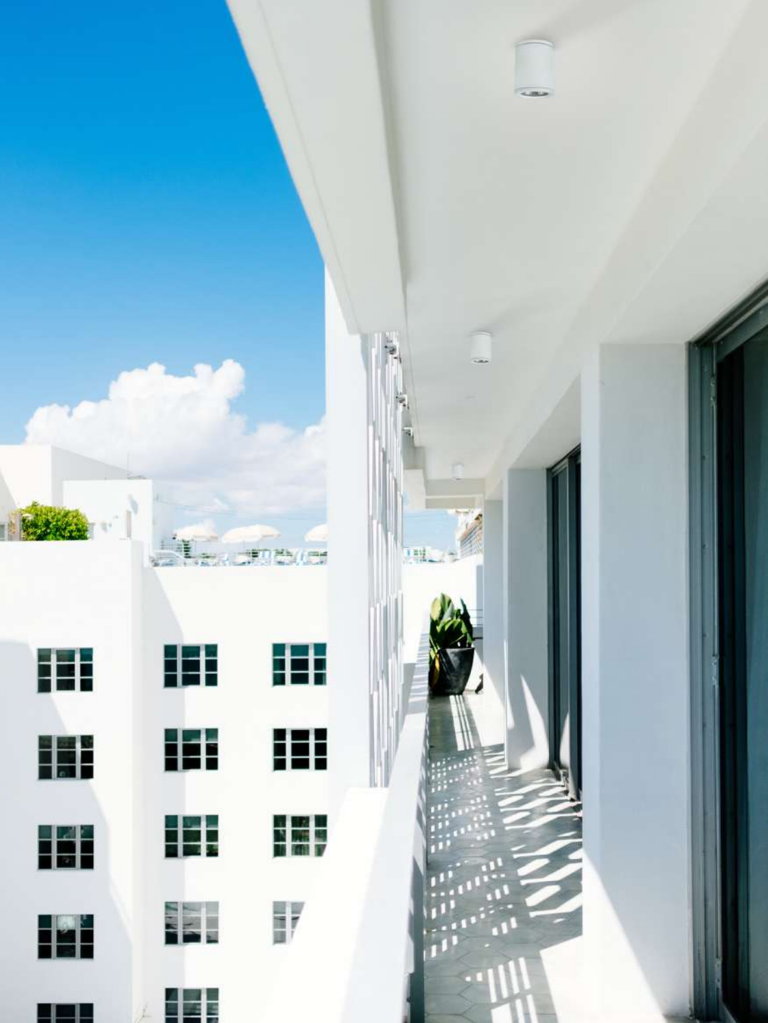
OUTDOOR - CEILING FIXTURES
