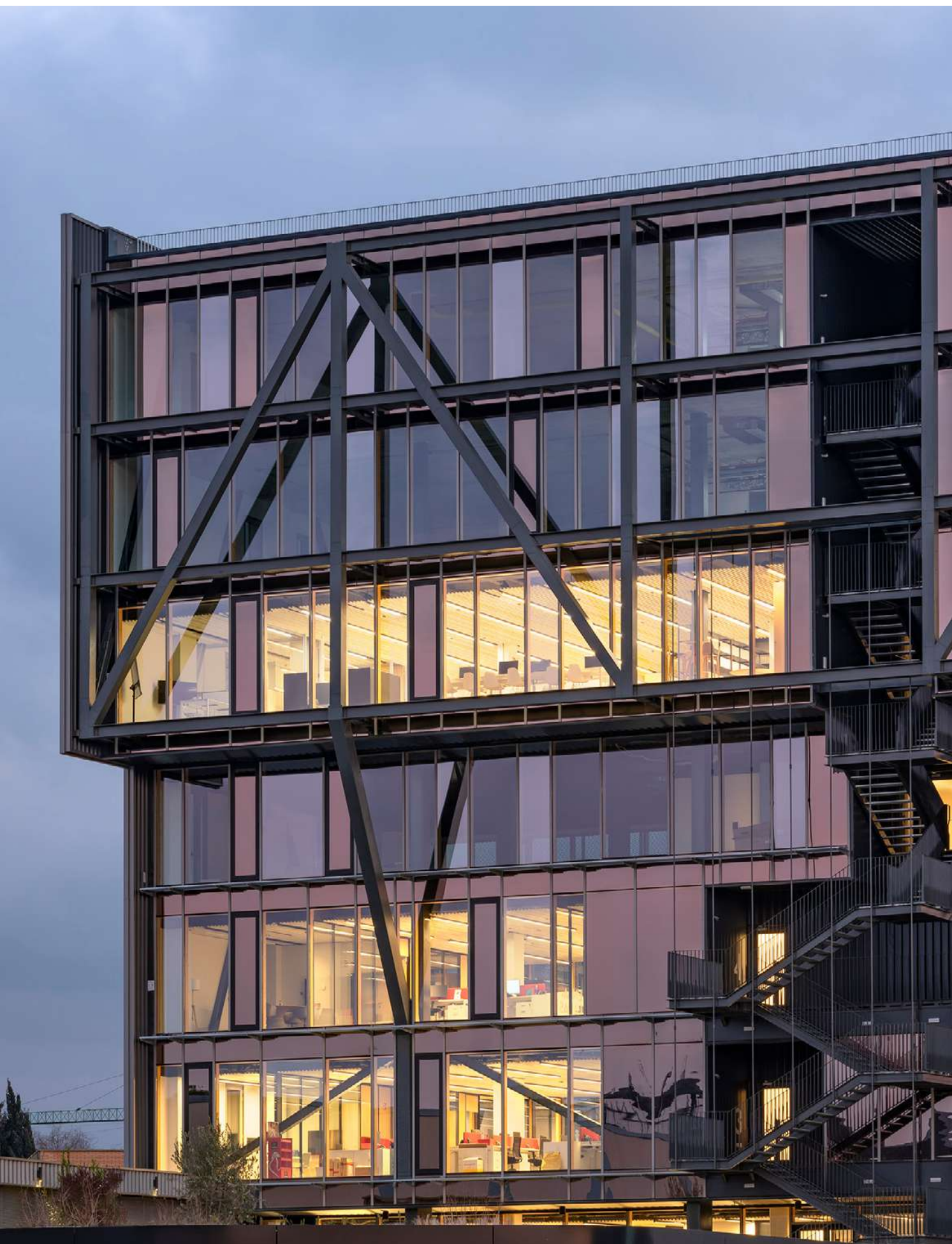
SLOW BUILDING, BARCELONA (SPAIN) Architecture: Ballo Rull
